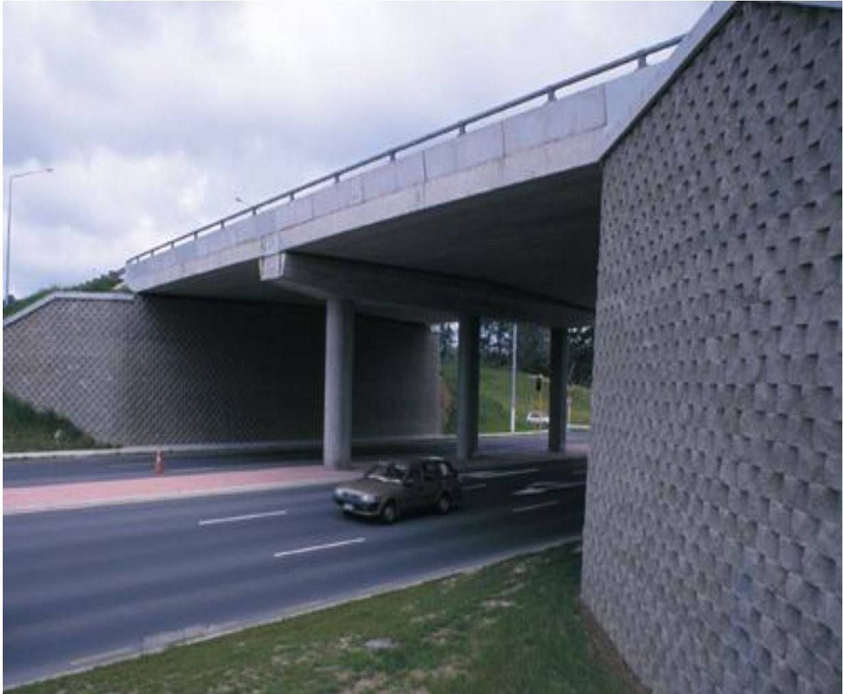
VE ALTERNATIVE 6 WITH MODULAR BLOCK WALLS
