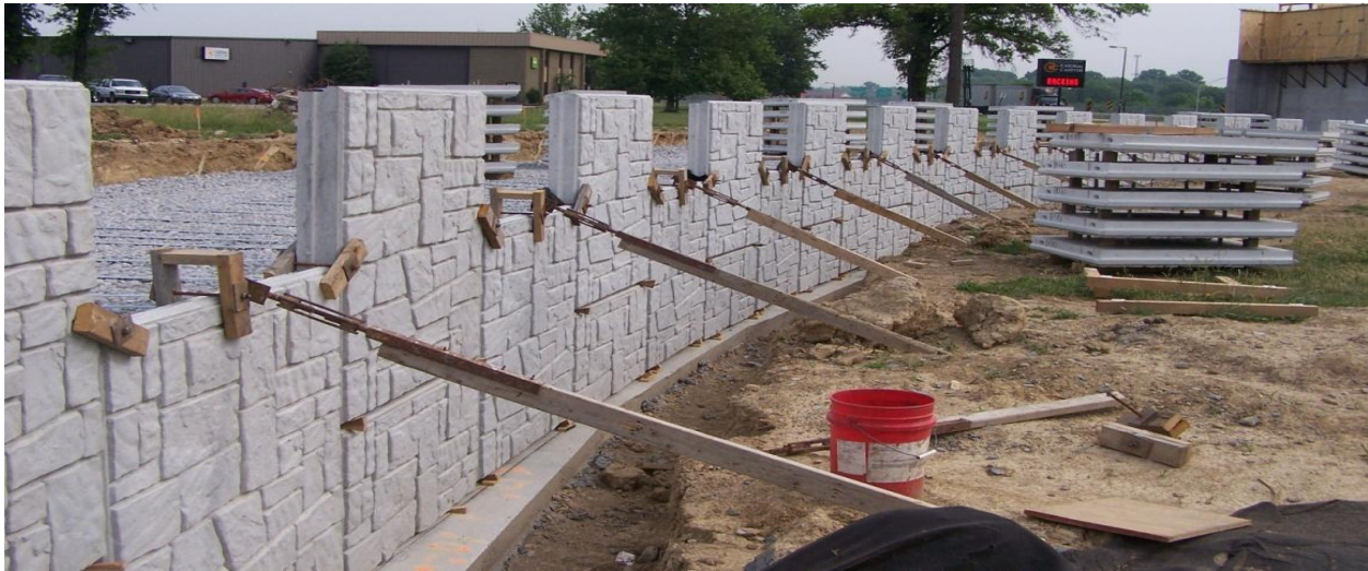
CONSTRUCTION OF MSE WALL
