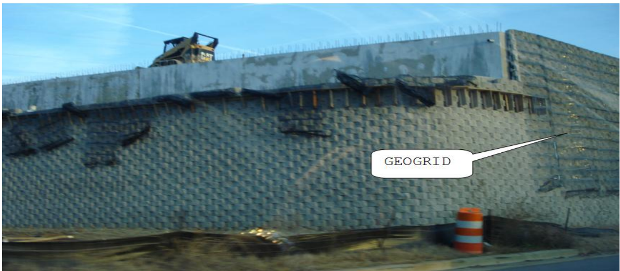
MODULAR BLOCK WALL UNDER CONSTRUCTION
