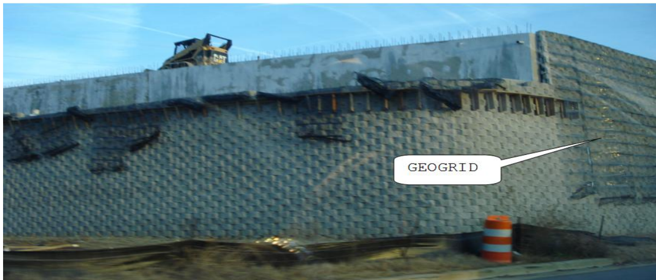
MODULAR BLOCK WALL UNDER CONSTRUCTION
