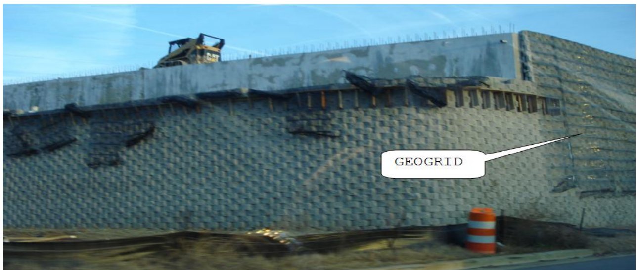
MODULAR BLOCK WALL UNDER CONSTRUCTION
