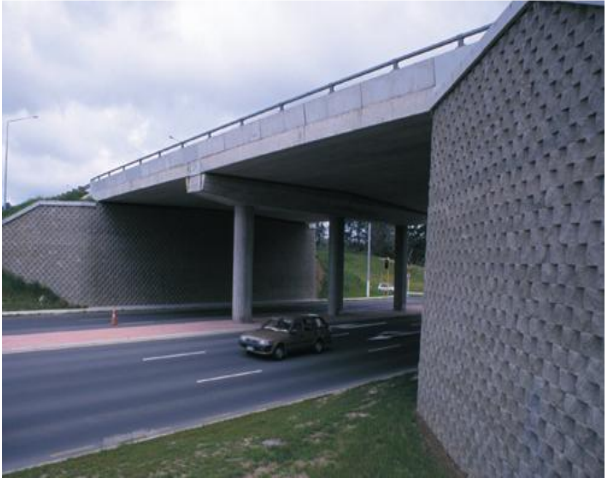
VE ALTERNATIVE WITH MODULAR BLOCK WALLS
