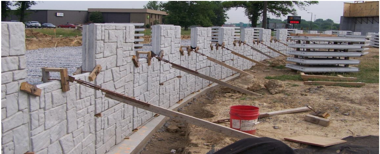
CONSTRUCTION OF MSE WALL
