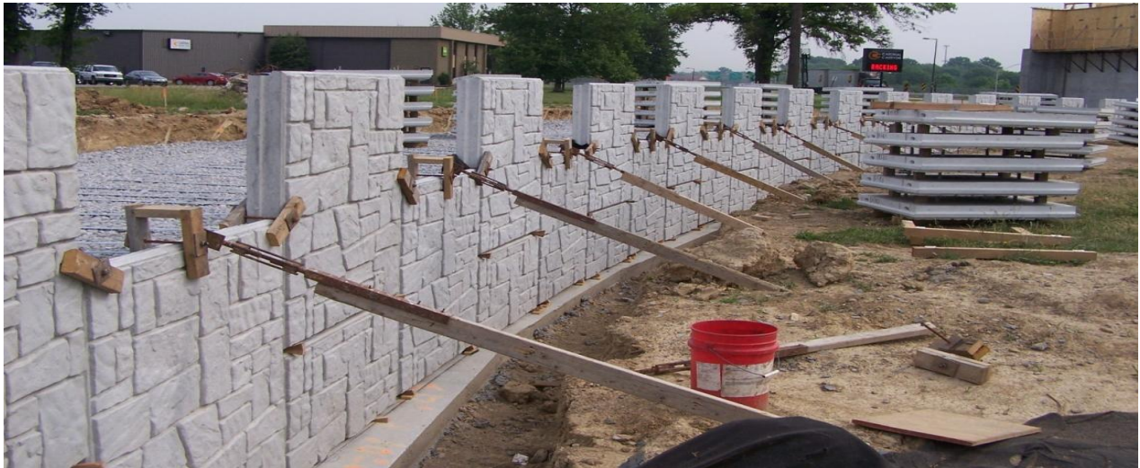
CONSTRUCTION OF MSE WALL
